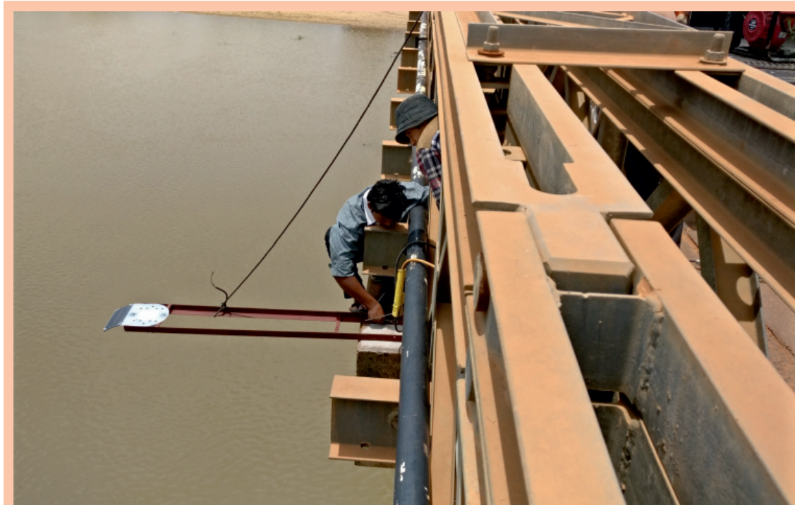
Picture 2: Installation of a PIN-developed automated gauge to a bridge
